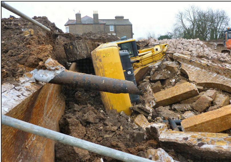
**Failure to fully assess the changing ground conditions on this site allowed the excavator to overload a barrel vaulted brick structure which collapsed causing the machine to fall through.**
